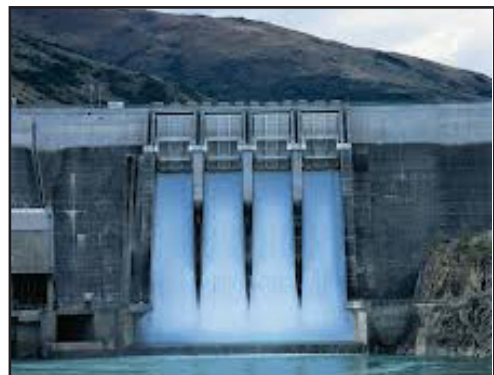
Hydro Electric power
