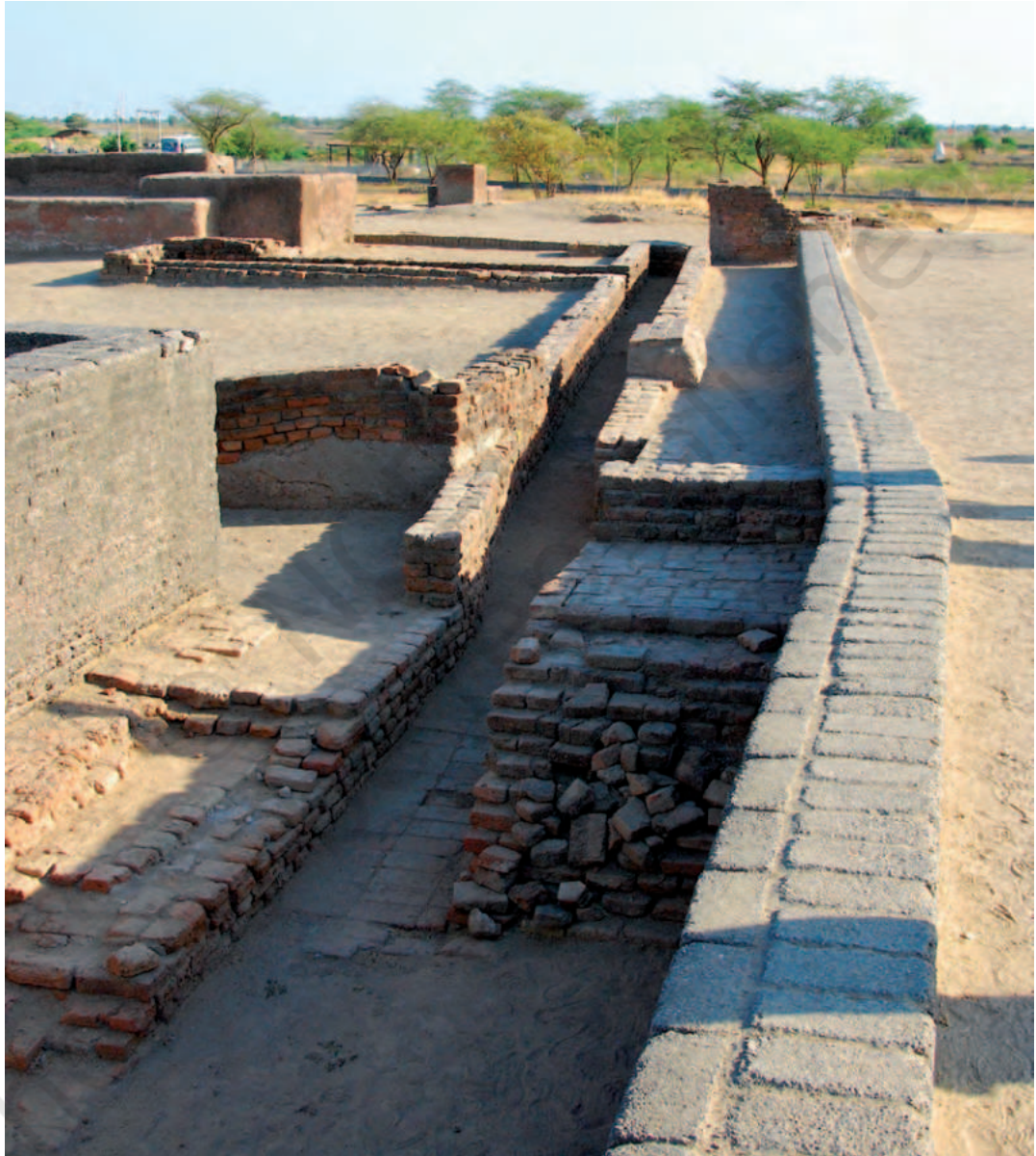
Fig. 6.7. Drainage system at Lothal (Gujarat)
