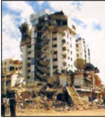
Fig. 3.3a: Destruction caused by an Earthquake in Gujarat
