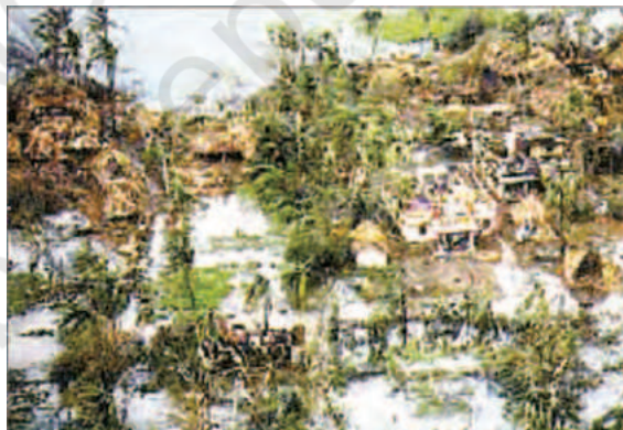
Destruction caused by a cyclone
