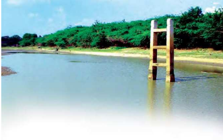
Fig. 5 A ninth-century sluice gate in Tamil Nadu. It regulated the outflow of water from a tank into the channels that irrigated the fields. A sluice gate is traditionally a wood or metal barrier which is commonly used to control water levels and flow rates in rivers and canals.
