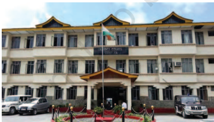
District Courts Complex in Namchi, South Sikkim http://districtcourtsnamchi.nic.in
