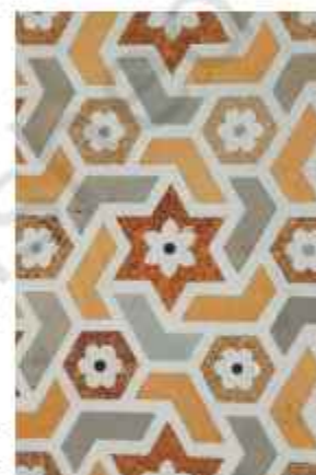
Dado panel on the wall, Agra
