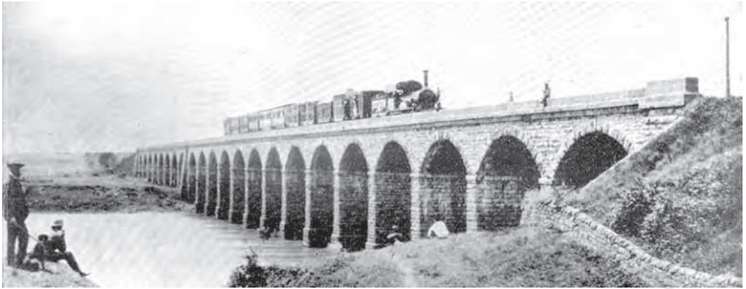
Fig. 1.4 First Railway Bridge linking Bombay with Thane, 1854
