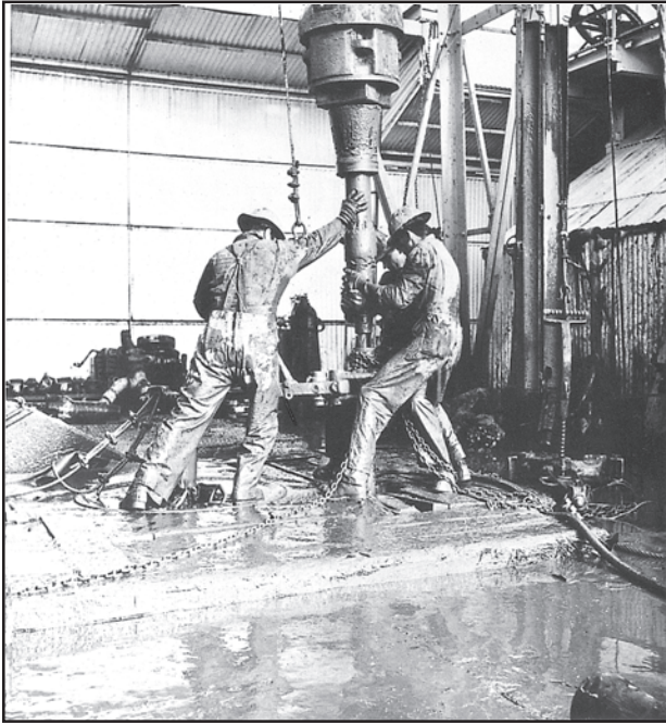
Fig. 4.18: Oil drilling operation in the Gulf of Mexico
