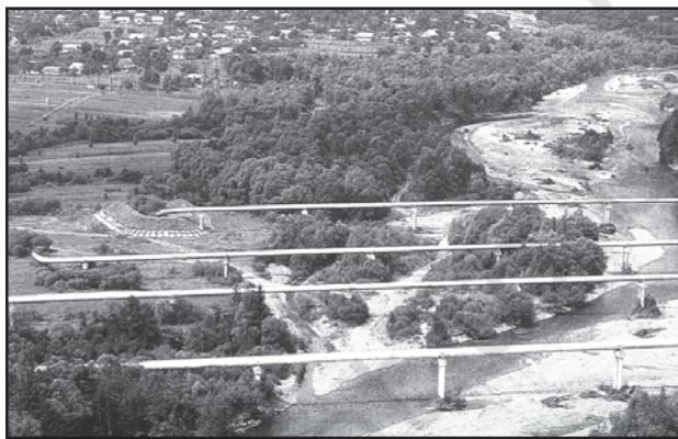
Fig. 7.17: Pipelines transporting natural gas in Ukraine
